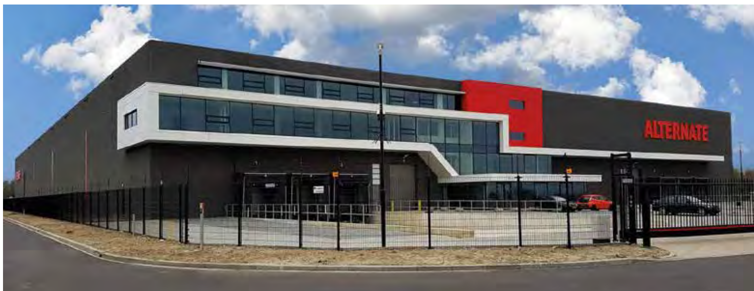
Alternate, full electric energieneutraal distributiecentrum.
