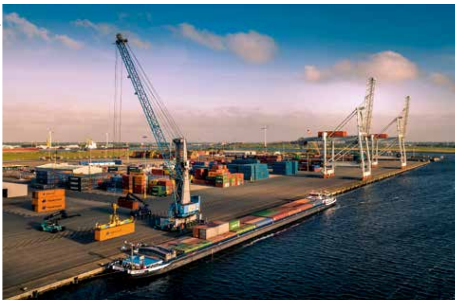
TMA Logistics Terminal Amsterdam.
